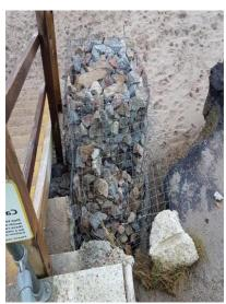
In 2024, despite the installation of additional gabion baskets, the extensive erosion beneath and around the lower steps and structural supports necessitated an emergency response to remove them.
